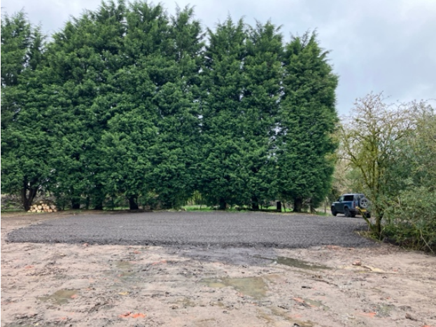
Car Park Area
